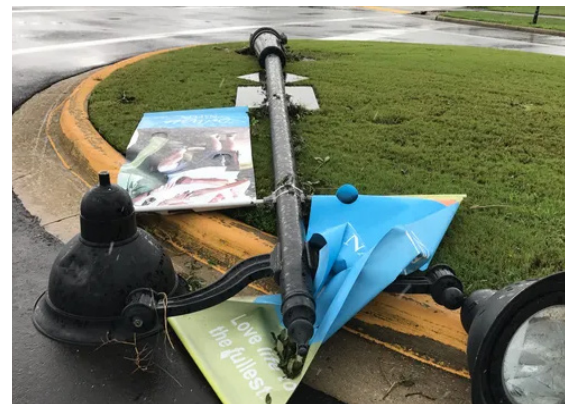
Static brackets can cause significant wear on banners, brackets, and poles, leading to liabilities and hazards.
